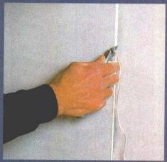
To make butt seams as flat as possible, both edges are trimmed back on a slight bevel to remove loose paper before the drywall is installed.
