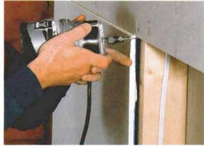
**Seams all right to me.** As an alternative to cutting a small rip, a sheet that's too large for its intended space is allowed to lap over the adjacent sheet and trimmed using its underlying neighbor as a stencil.
