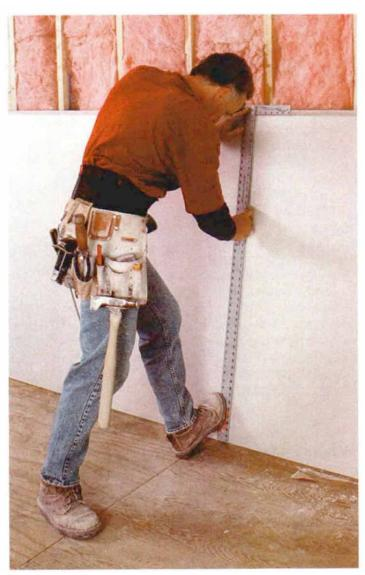
"Score and snap" is not a wrestling move. The author uses his left hand and foot to steady the 4-ft. drywall square, which serves as a straightedge for crosscuts (photo left). After scoring the face and breaking the gypsum core, he makes a foot-long cut through the back paper (photo right) before snapping the sheet in two (photo left, facing page).
